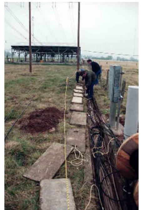
some reason the rodents found the pipes and cable covering edible and they chewed contentedly, eventually causing shut-downs. These manifested themselves when array switches refused to operate, the revertives disappeared or the air compressors supplying the field overheated.
